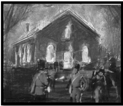
The Burning of the Courthouse in Tappahannock
